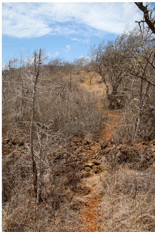
Footpath going up the Seru di Warawara (Warawara hill) at Santa Cruz, Curaçao, at the end of a long period of drought (24 May, 2014). In the picture a low dam running across the hill can be seen. Such structures are called "faha" meaning belt. Many were constructed in the past to conserve run-off rainwater, forcing the water into the ground, and also to a lesser extent to combat erosion.
