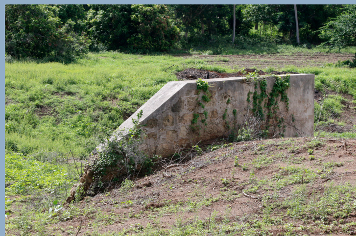
Masonry protection of dam ends. Usually the dam ends are protected. Larger dams also have overflow structures.
