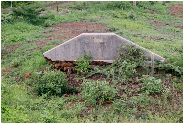
Masonry protection of dam ends. Usually the dam ends are protected. Larger dams also have overflow structures.
